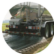
Dust treatment for dusty roads
